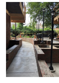
East Tower Ramp Up!
