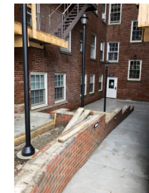
East Tower Ramp Down
